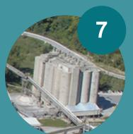
DISTRIBUTION From the grinding mills, the cement is conveyed to silos where it awaits shipment. Cement is shipped by trucks, rail, or barge.
