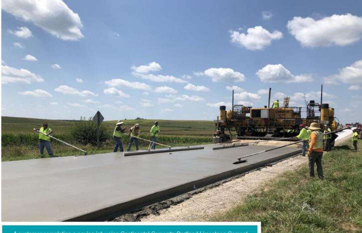
A customer completing a paving job using Continental Cement's Portland Limestone Cement
